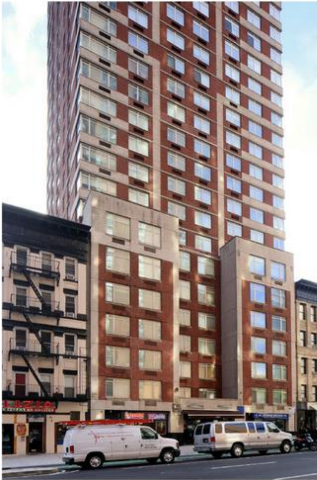
MANHATTAN Chartwell House on Second Avenue was appealing. But apartments there also were too expensive. Susan Fisher Plotner for The New York Times
